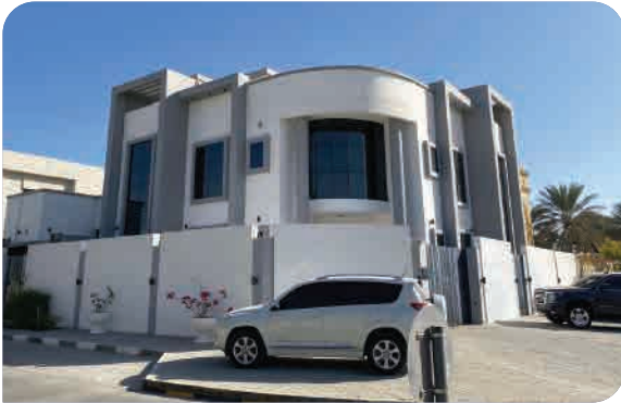
G+1 Villa Al Khuwair, Kalba Design, Construction
