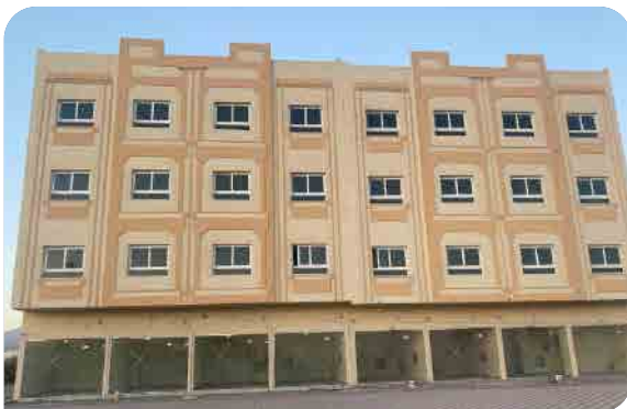
G+3 Terjaria Soor, Kalba Design, Construction
