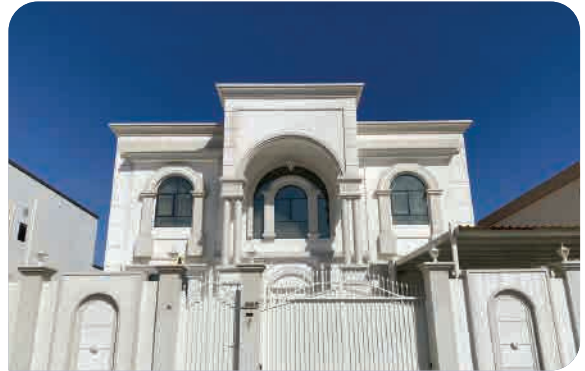
G+1 Villa Al Saaf 6, Kalba Design, Construction
