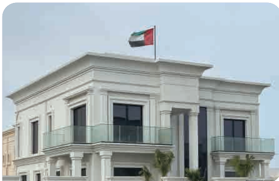
G+1 Villa Al Ghail 4, Kalba Design, Construction
