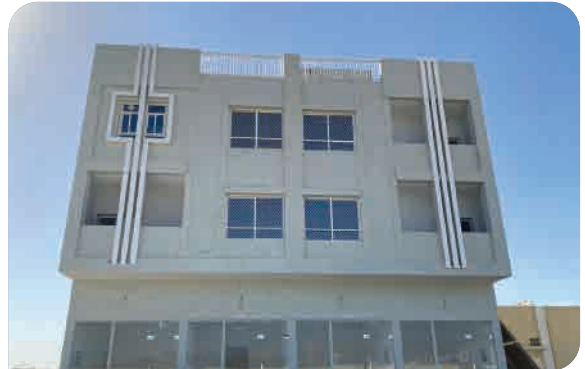
G+2 Terjaria Soor, Kalba Design, Construction
