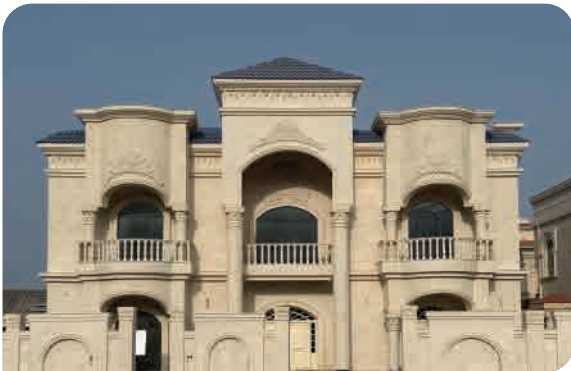
G+1 Villa Al Ghail 3, Kalba Design, Construction
