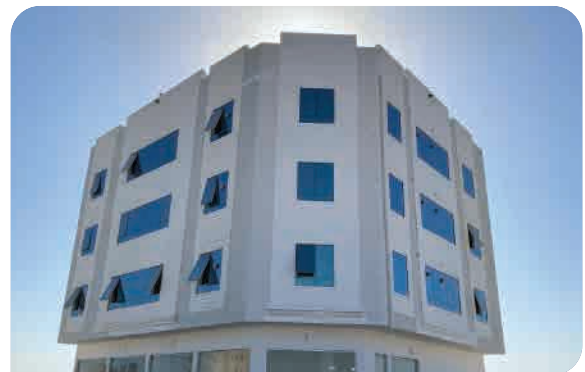
G+3 Terjaria Soor, Kalba Design, Construction
