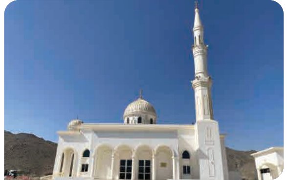
350 Capacity Masjid Al Ghail 3, Kalba Design, Construction
